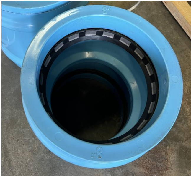
Figure 2-7 Reiberlok gaskets were installed into the sleeve joint
