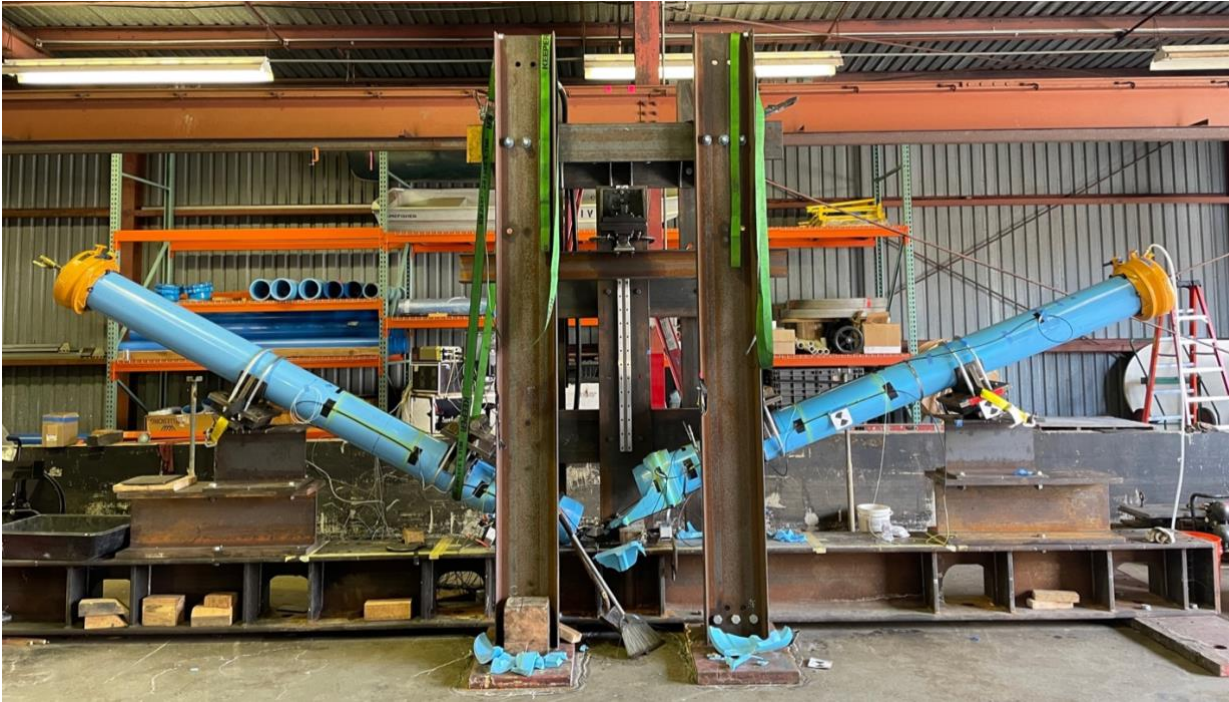
(a) Overall failure
