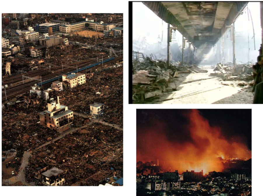
Figure 11. Fire Spread Damage in Kobe City after 1995 Kobe Earthquake.
