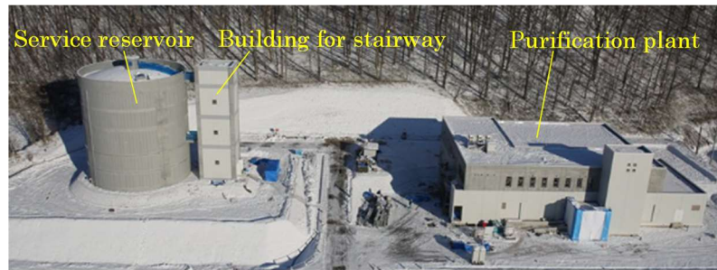
Photo 7. Tomisato purification plant and service reservoir before the earthquake. (Maruhironozawa Co., Ltd., 2018)
