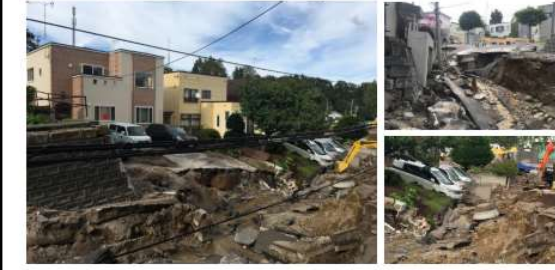
Liquefaction, 2018 Hokkaido Eastern Iburu earthquake
