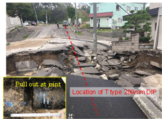
Photo 6. Damage to 200 mm-diameter pipe.
