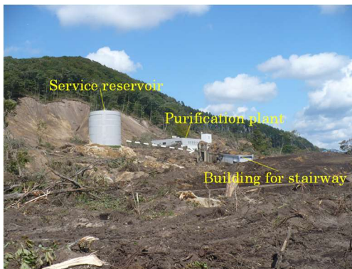
Photo 8. Tomisato purification plant and service reservoir after the earthquake. (Geographical Survey Institute, 2018)
