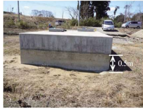
Fig. 27 五本松第1分水工の浮上 Uplift of Gohomatsu No.1 division works
