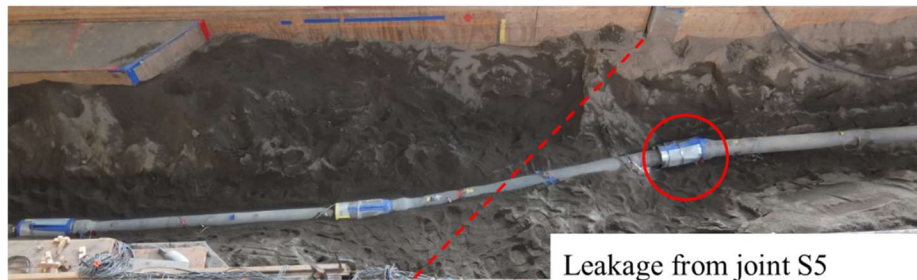
Photo 9. Test specimen after the test
